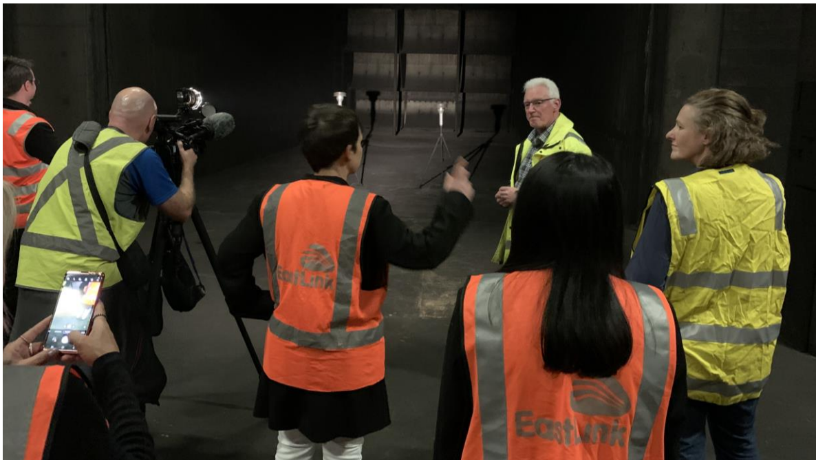
Image 10: Stakeholder tour with the Minister for Roads and Road Safety, The Hon. Jaala Pulford (centre) in the tunnel ventilation facility (22 February 2020)
